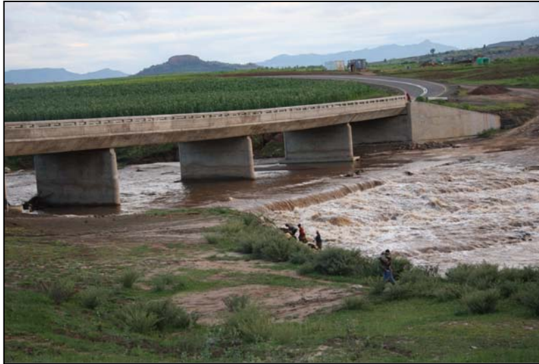
Bridge 1 on the Phuthiatsana River - Ha Makhoathi
